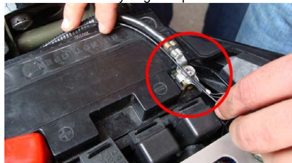
Figure 12: ground cable correctly connected.
